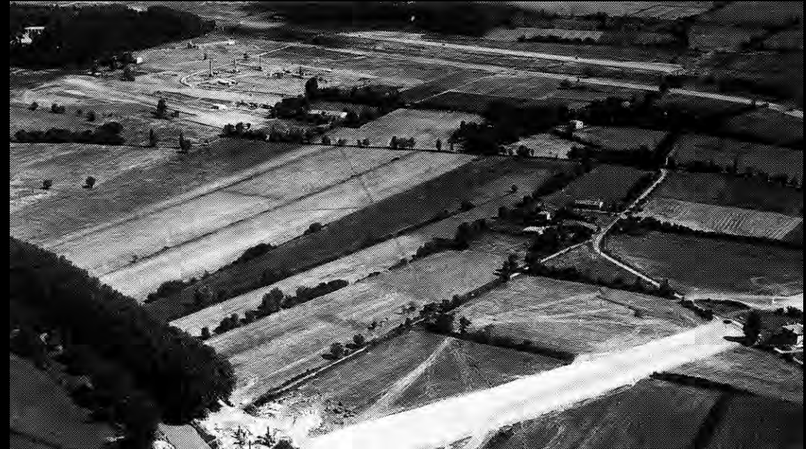
The CST before work started
